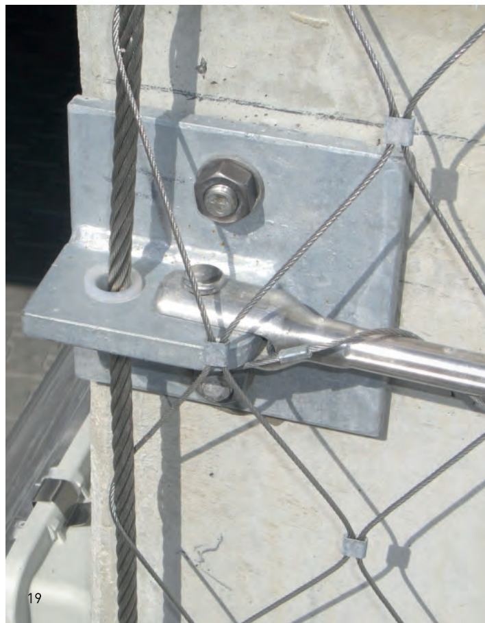
16 Netz vor Pfostenebene an Randseilen Mesh in front of post plane with border cables
